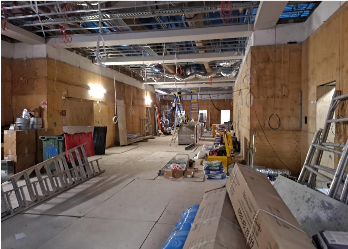
Figure 3: Existing internal entry hall
