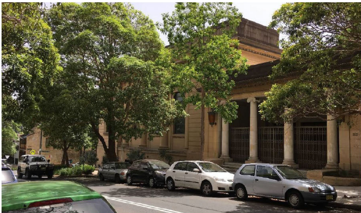
Figure 2: Site, prior to works commencing, viewed from Liverpool Street
